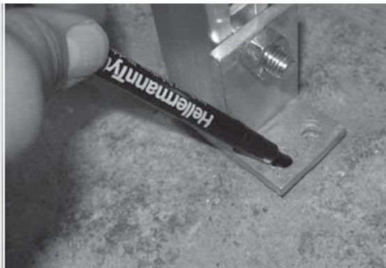
Fig 5.1.15 After completing the holding rack, you have to anchor it on the bottom. For doing that, you have to mark on each T-piece two boreholes. You have to move the rack aside and the boreholes have to be made by a 12 mm masonry drill bit. Following the 12 mm plugs have to be inserted in the holes, the rack has to be centered on the boreholes and it has to be bolted on the bottom with the 8 x 60 mm -screws.
