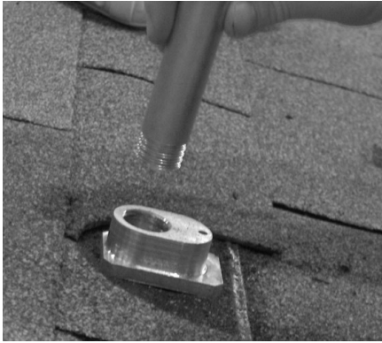
Fig. 4.2.6 Thread post into base. Using the adjustable pliers, tighten post into base by turning clockwise.
