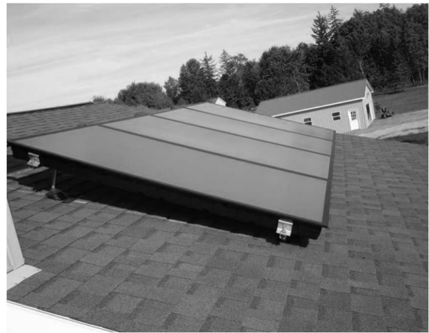
Fig 5.1.18 The lateral attachment clamps have to be fixed by M10 x 30 bolt, u-washer and nut in the lateral long hole of the horizontal rail.
