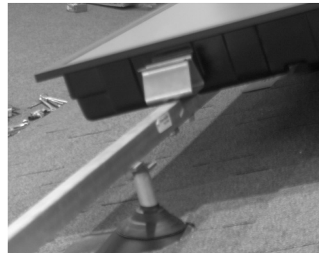
Fig 4.2.25 Slide Heliostar panel on rail using indents provided on back of panel until the anchor point meets the center bracket. If necessary make adjustments on offset brackets to square up panels.
