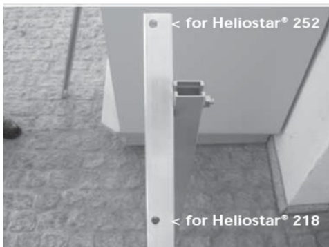
Fig 5.1.9 Important: For the installation of horizontal rails you will find pre-installed holes. In the upper area of the shown installation rails there are 2 holes, the upper holes are to position the horizontal rail for the installation of the Heliostar® 252
