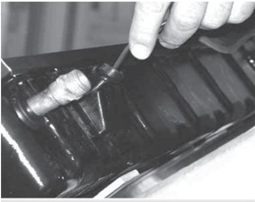
Fig 4.2.27 Remove the grommet next to the pipe on the return of the collector field and slide it over the cable of the temperature sensor: insert temperature sensor into the immersion sleeve as far as possible and remount the rubber grommet in the collector.
