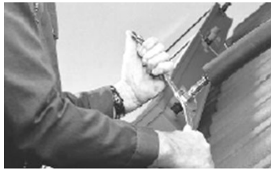
Fig 4.2.29 Use the supplied gasket and two wrenches to tighten the fitting. Repeat process as necessary. Use of a single wrench will cause internal damage to the collector piping.
