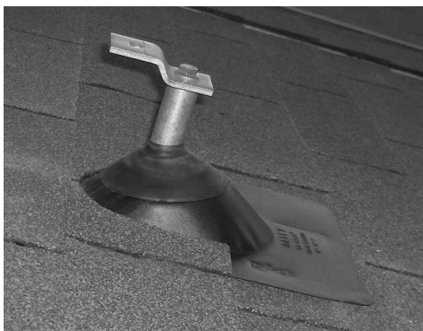
Fig. 4.2.11 Repeat the procedure for the six required anchor points. The center brackets should be on 48" horizontal centers. The last set of brackets should be on 24" centers or 32" centers (horizontal) depending on the rafter centers. The Roth frame will not accommodate a 48" on center configuration for the final set of brackets. The combination of the offset brackets and the unique adjustability of the horizontal rail will allow for this combination.
