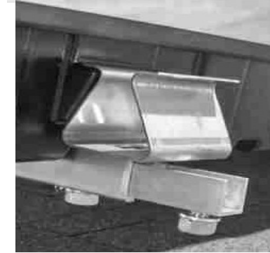
Fig. 4.2.18 Center panel anchor bracket
