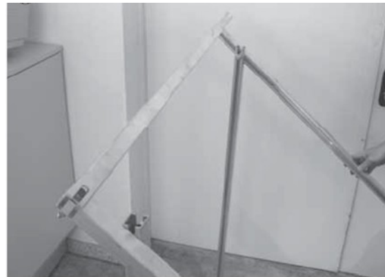
Fig 5.1.11 The distance of the outer edge slope rail compared to outer edge horizontal rail should be 2 15/16" (75 mm).
