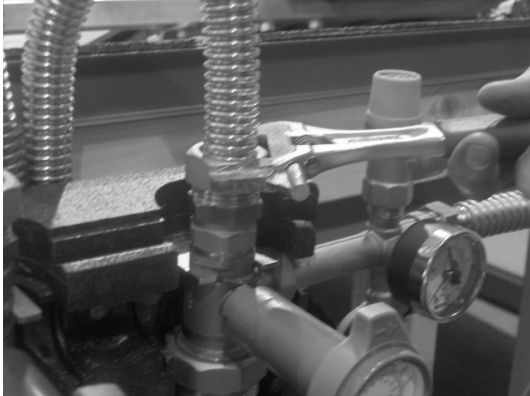
Fig 6.0.11 Connection using Roth basic fitting set for 2 in 1 flexible tube. This is the 3' flexible pipe from the collector to the 2 in 1 pipe. The adaptor (above) goes from the DN 20, 2 in 1 pipe to the G 3/4" connection on the pump station.
