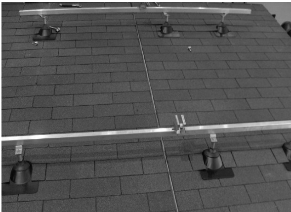
Fig 4.2.23 Finished roof rack for two panel array
