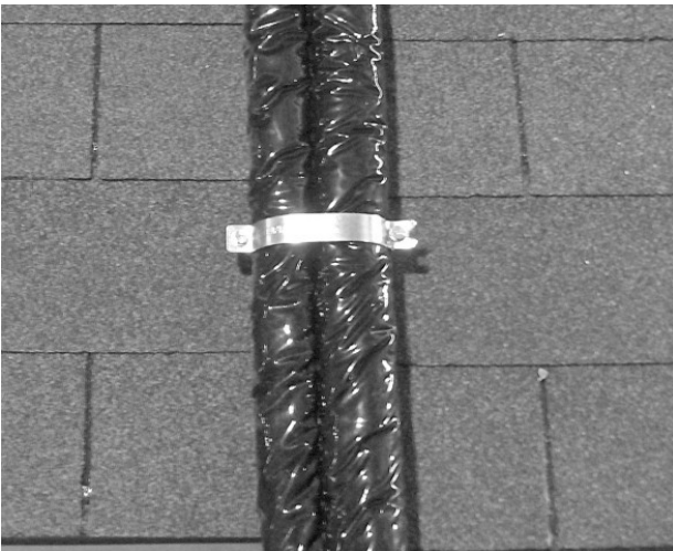
Fig 6.0.7 The integral insulation of the 2 in 1 piping system prevents heat losses on the roof and in the attic spaces.
