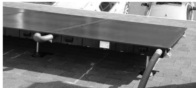
Fig 4.2.30 We have completed the basic roof installation. Now we must determine how we are to get our solar piping to the mechanical space. This can be as simple as running Roth 2 in 1 piping down the side of the roof and through the wall into the mechanical room, another penetration through the roof with flashing. Whatever is the least evasive piping requirement and still meets our customers required aesthetics.
