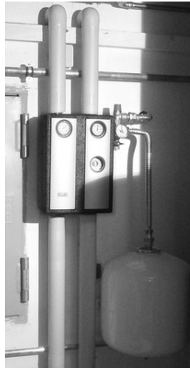
Fig 6.0.14 Roth Solar Pump Station Shown with completed piping and expansion tank
