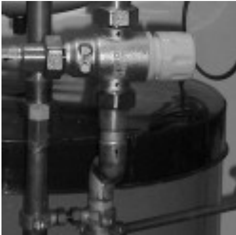
Fig 6.0.11 installation of anti-scald device on the storage tank is recommended. potentially high domestic water temperatures involved with solar systems could cause a possible safety issue.
