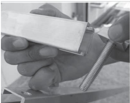
Fig 5.1.10 The horizontal rails are inserted with M10 x 60 screws in the U-shaped cut and completely pushed in the installation rail.
