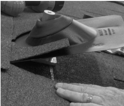
Fig. 4.2.8 gently lift shingle and slide flashing over the post and up under shingle. It may be necessary to use a putty knife to break the adhesive bond on the back of shingle to allow for the insertion of the flashing.
