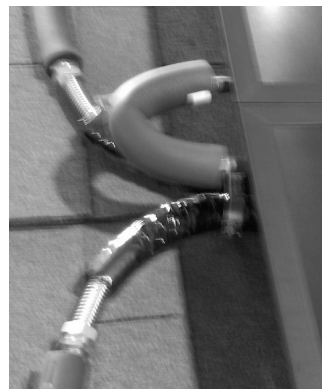
Fig 6.0.5 the solar panel flexible piping connected to the 2 in 1 piping.
