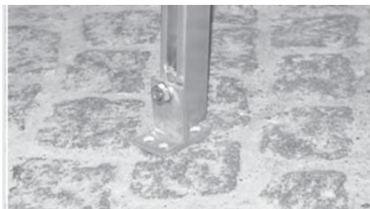
Fig 5.1.7 The prepared connection is inserted in the installation rail and afterwards fixed to the anchor. This procedure is carried out on the lower end of the vertical and slope rail.
