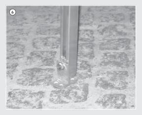
6. The prepared connection is inserted in the installation rail and afterwards fixed. This procedure is carried out on the lower end of the vertical and slope rail.
