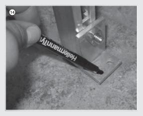
14. After finishing of the holding rack, you have to fix it on the bottom. For doing that, you have to mark on each T-piece two boreholes. You have to move the rack aside and the boreholes have to be made by a 12 mm rock drill. Following the 12 mm plugs have to be inserted in the holes, the rack has to be posed on the boreholes and it has to be fixed on the bottom with the 8 x 60 mm wood-screws.
