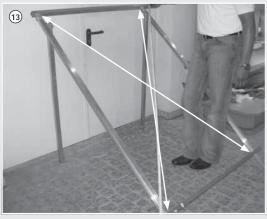
**13.** To be sure that both horizontal rails have the same distance you have to find out the diagonal distance.
