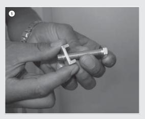
2. Attach with washer and nut to vertical installation rail. (Insert until end of long whole)
