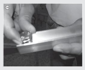
**19.** Both M12 x 20 screws have to be inserted in the connection rails for the upper and below horizontal rail as shown on the photo.
